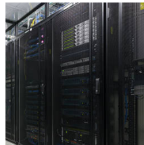
Uninterruptible Power Supply
